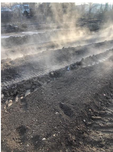
Exothermic reaction taking place during a drying process on a very wet site. Steam rising from the soil
